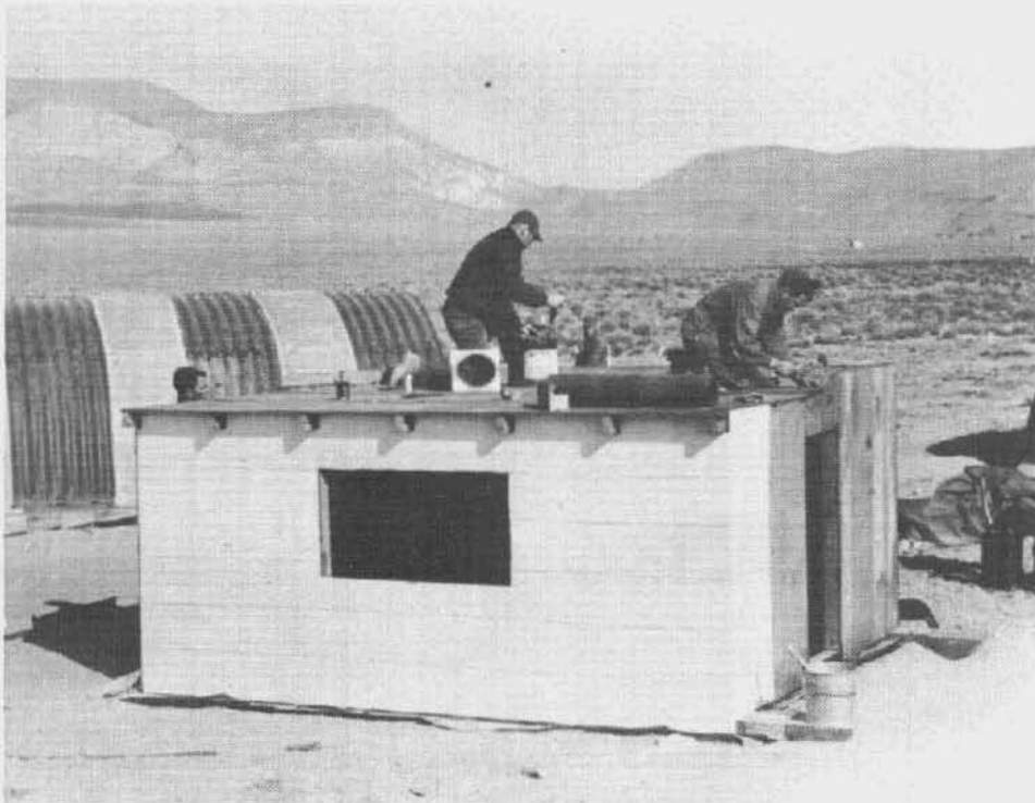
Fig. 6.3 Preparing the Building Surfaces
